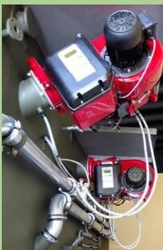
An automated burner serves for the heating of the combustion chamber subject to the temperature of the fire room. For heating the unit at start up the burner is in operation.
